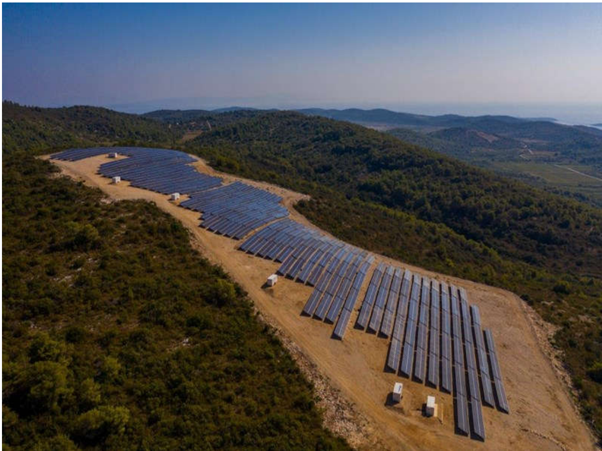
Figure 1 Solar power plant Vis, island of Vis, Croatia
